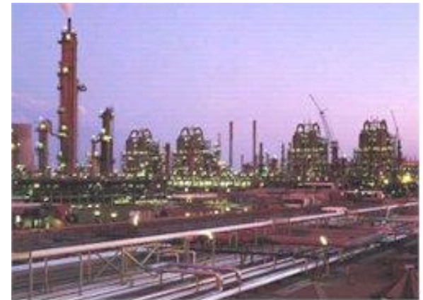
CTL facility at Secunda. Source: www.scienceinafrica.co.za
