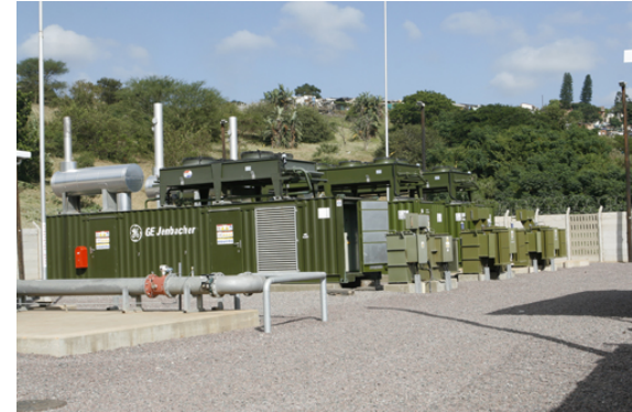
The landfill gas to electricity generation plant at Durban eThekweni . Source: www./impumelelo.org.za/
